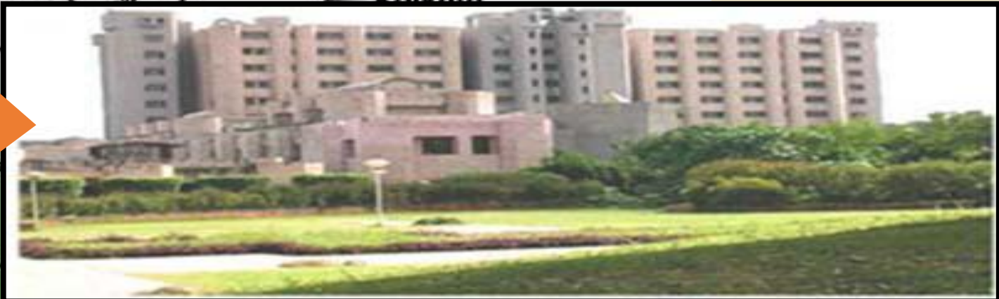
Sanjay Gandhi Post Graduate Institute of Medical Sciences (SGPGIMS) Tertiary Care Supespecialty Hospital
